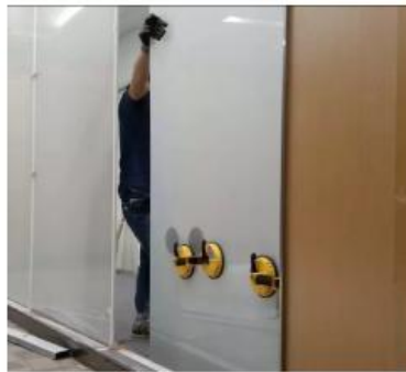
Glass vertical installation
